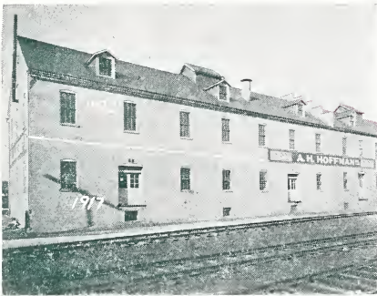
Additions to Original Warehouse.
